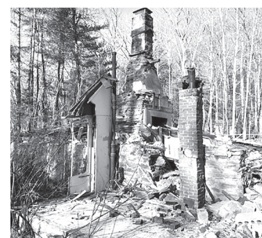
Photo by John Talley Crews demolished the home on Thursday, February 8.
