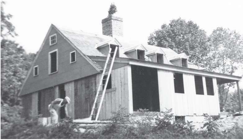
The back of the house under construction. Note the pine tree at the chimney, placed during a traditional “topping out” ceremony after the roof beam is put in place.
