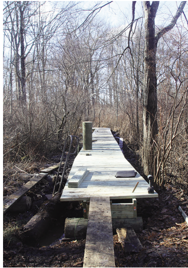
The new boardwalk, a work in progress.
